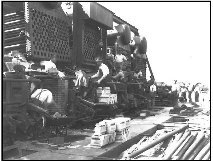
Boiler Brickwork for the Fire Box
