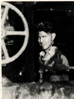
Dubbs coke handler at work on steam and water manifold.
