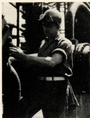
Hard at work on after-coolers of plant's coker and reformer section.
