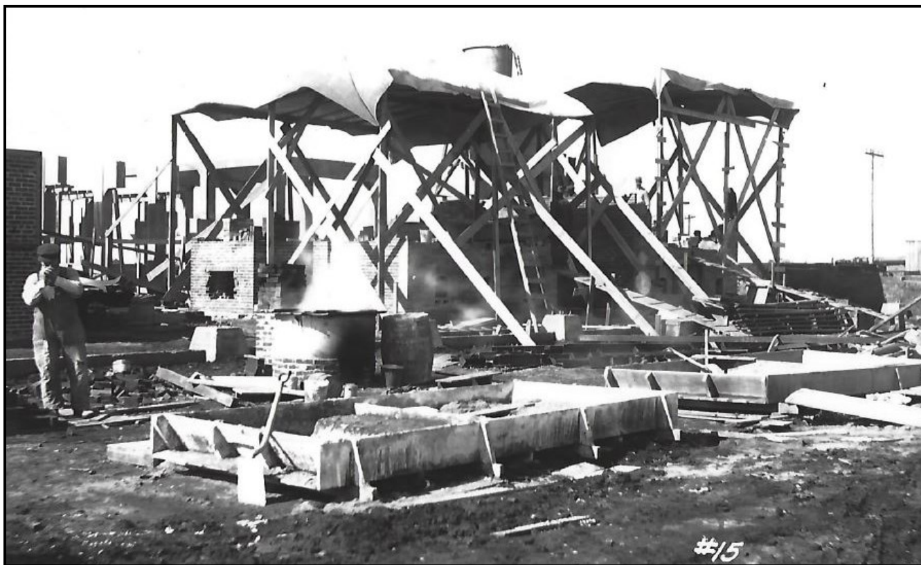
Trumble Unit Heater Brickwork
